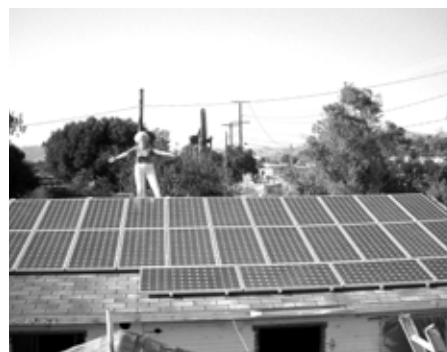
Jan doing a sun dance over the solar collector panels.
